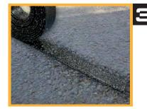
Remove the packaging and carefully place the overbanding tape on the road surface with the top facing up. Position the tape as accurately over the crack for optimum performance. Cut to size.
