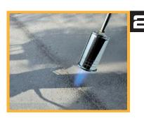
Using a suitable propane torch, remove all moisture present (if any) and preheat the area prior to treatment.
