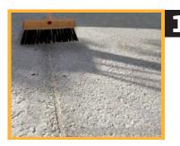
Prepare application area thoroughly by removing all sand, dirt, chemicals and oily substances.
