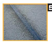
Leave the overbanding tape to cool and harden for 15 minutes. When cool, examine the tape and test by trying to lift it using a metal spatula or knife. If areas do lift, repeat step 4.
