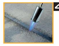
Heat the overbanding tape using a suitable propane torch, keeping the flame approximately 200-300mm from the tape. With a side to side motion, ensuring evenly distributed heat, heat the material gently until molten and it begins to bubble slightly and flow into the surface. Ensure both surfaces are fused together.
